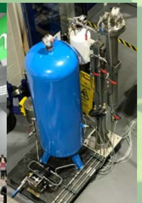
Task 1: Pressure unit under construction
